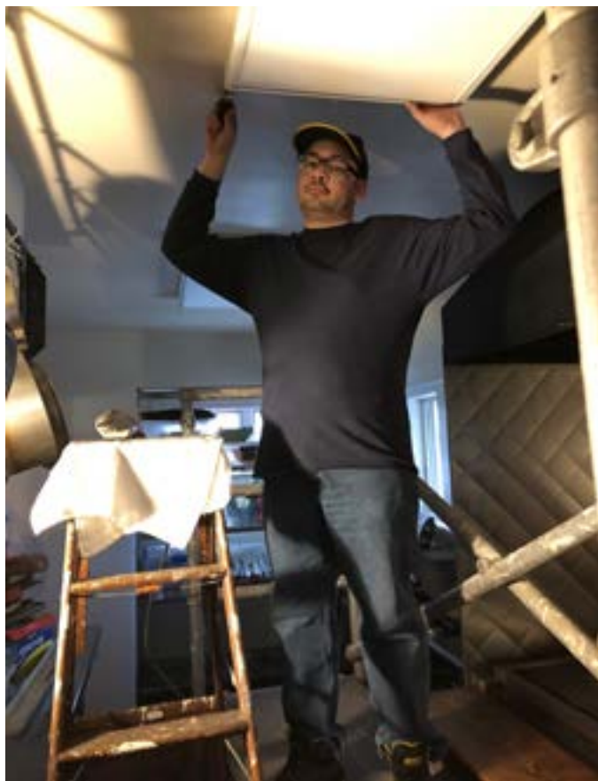
Christopher Hudson installing kitchen ceiling lights.
